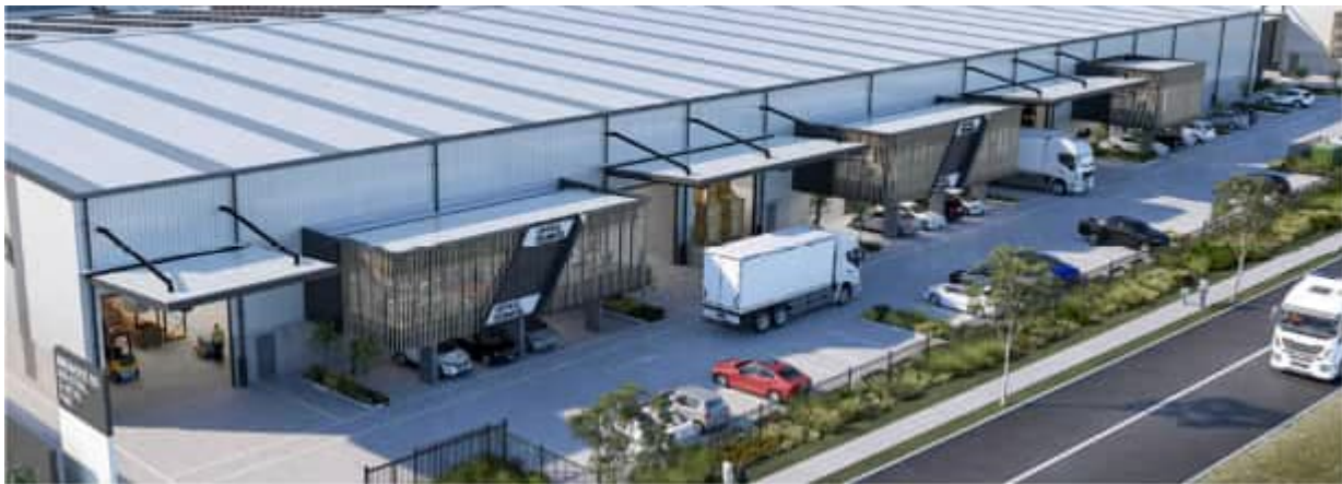
Figure 19 Indicative image of warehouses and ancillary offices
