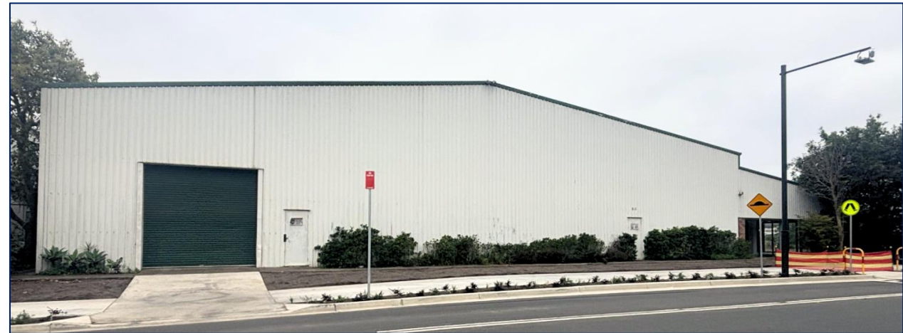
Lot 4B in Altitude Industrial Estate (top) and Site 611 (bottom)
