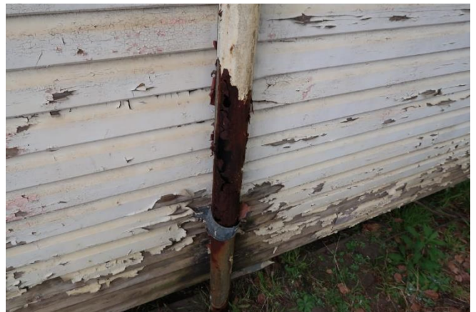
Corroded downpipe
