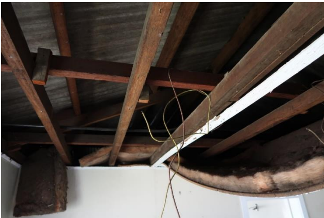
Timber framed roof structure
