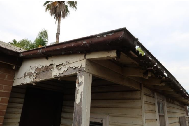
Corroded guttering
