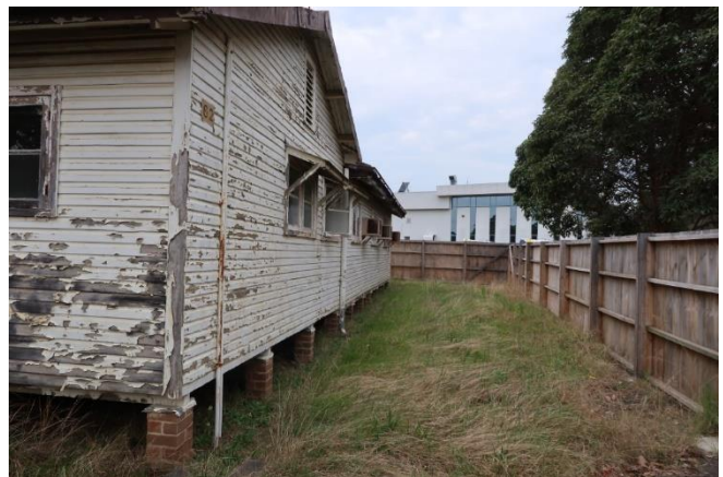
General view of external and perimeter fence
