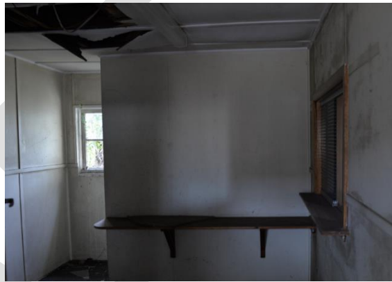
Figure 14. Reception room at Airport Avenue entryway.
