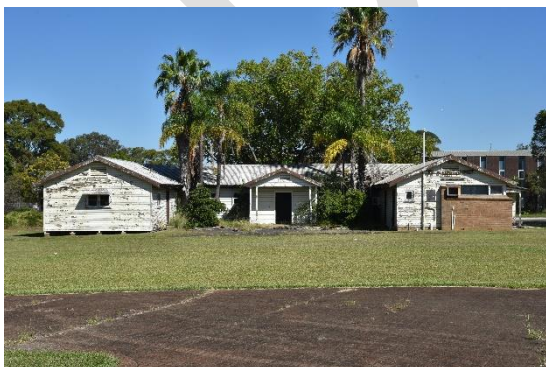
Figure 9. View west across former parade ground to the building's principal (east) elevation, showing palm tree plantings.
