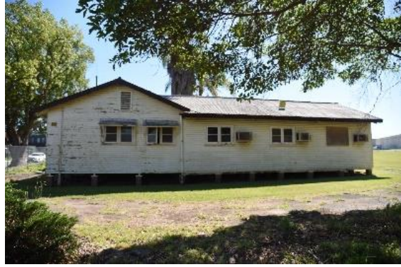
Figure 12. View of side elevation, looking north.
