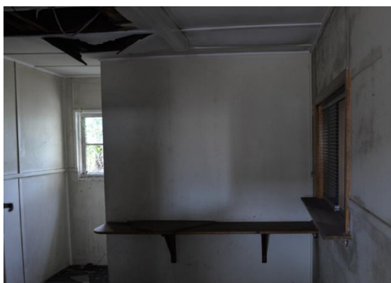
Figure 10. Reception room at Airport Avenue entryway.
