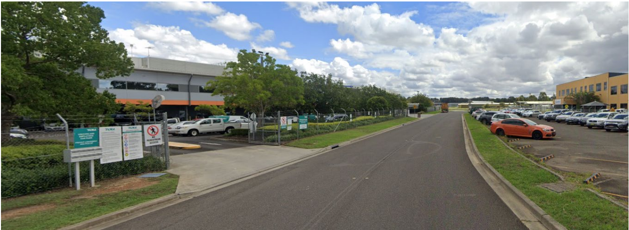
Figure 3: Nancy Ellis Leebold Drive (along site frontage looking north)
