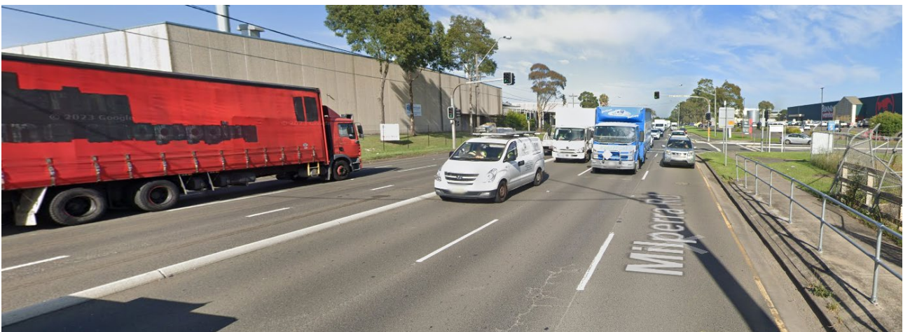
Figure 4: Milperra Road (looking west)
