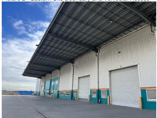
Picture 4 - Southern Warehouse Elevation
