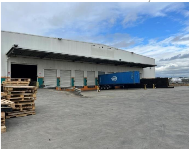
Picture 3 - Western Elevation of Warehouse
