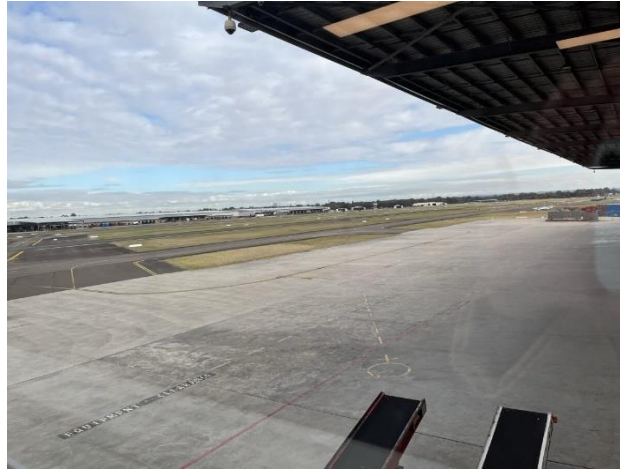
Picture 8 - Airport Apron Viewed Looking South East
