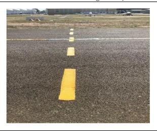
Manoeuvring Area Ground Marking This ground marking indicates the holding point into the manoeuvring area
