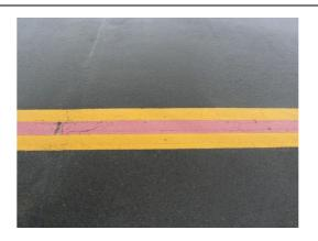
Aircraft Parking Limit Lines Yellow and red continuous line used to define an area in which the whole of a parked aircraft is to be confined.
