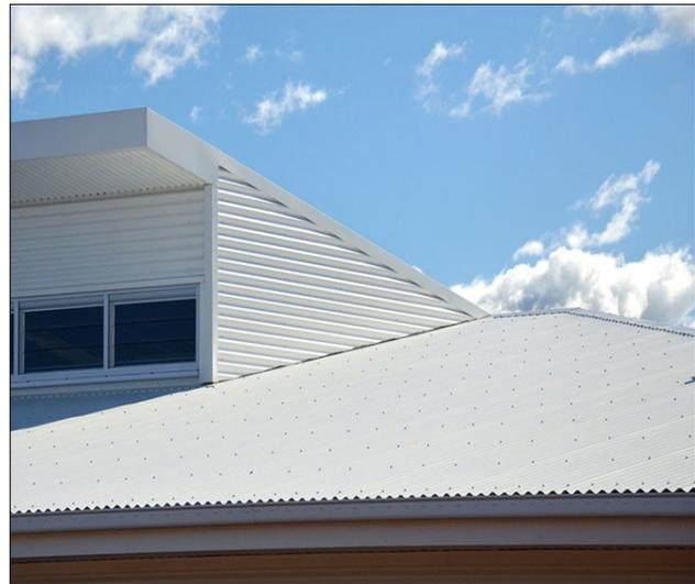
Figure 7 - Illustration of a light coloured (reflective) roof sheeting.
