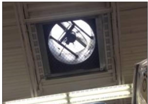
**Figure 10 - Motorised smoke exhaust fans can enable hot air to escape through roof, facilitating air ventilation.**
